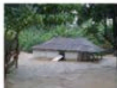
Roche a Bateau – private home flooded. Credit: Cote Sud Initiative
