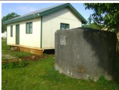
Example of house having a water tank without guttering
