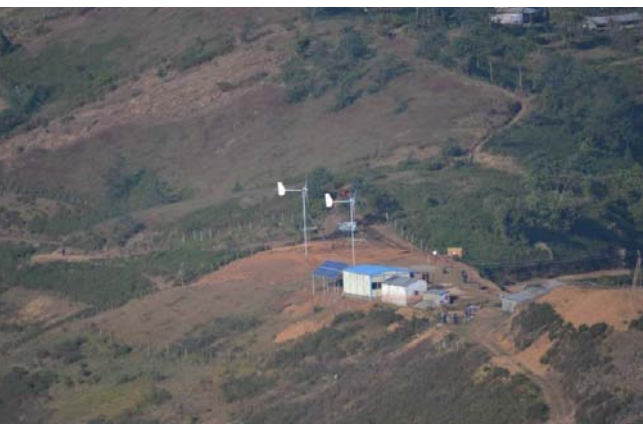
Small wind and solar hybrid renewable energy technology
