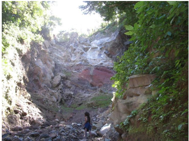
Figure 21: Landslide at falls of Baleine
