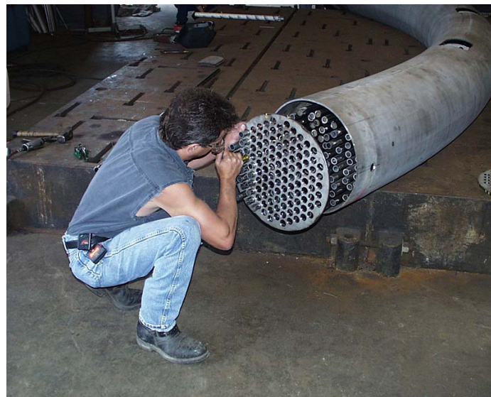
Figure 3: The “cheese plates” at the cradle ends with grout in the interstitial spaces between the individual sleeves hold the strands parallel to each other.
