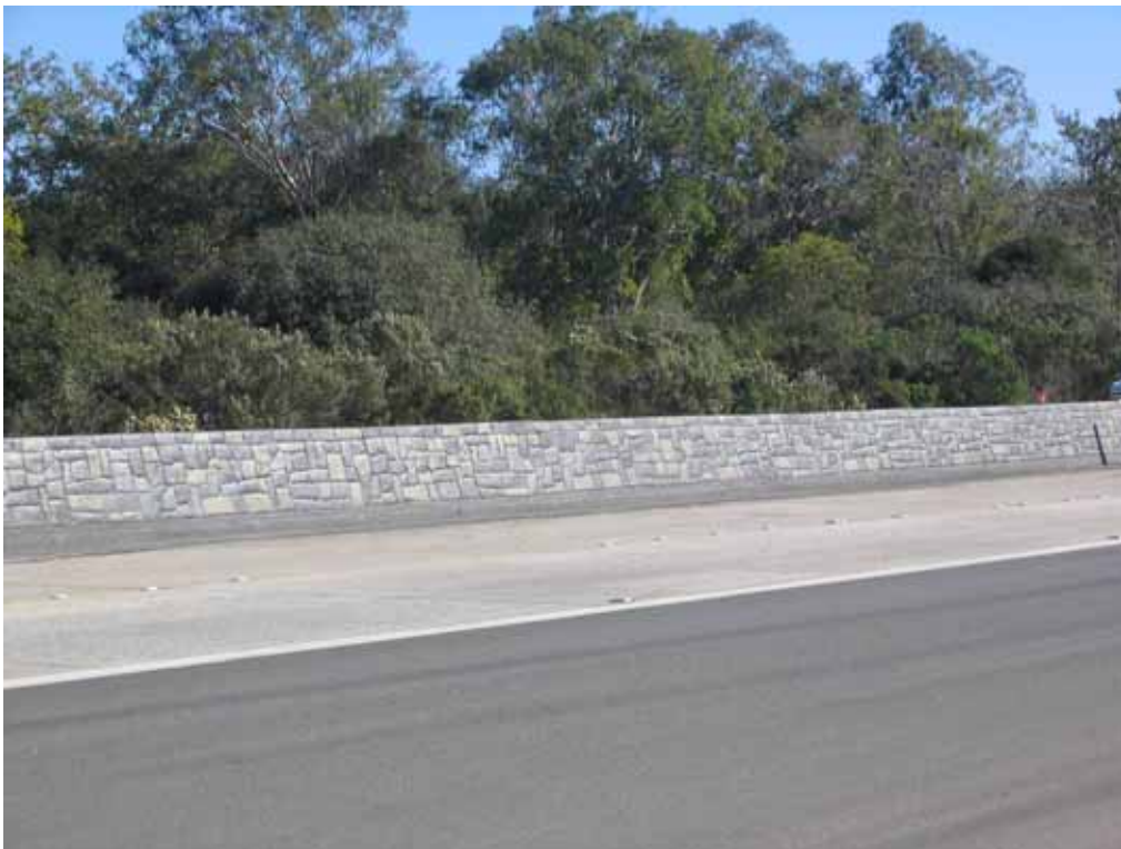
Median barrier on Hwy. 1 in San Luis Obispo, CA
