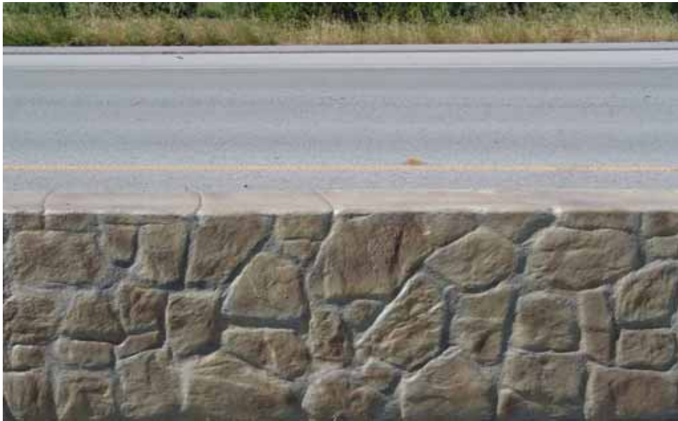
Median barrier on Hwy. 156 in Sa Juan Buatista, CA
