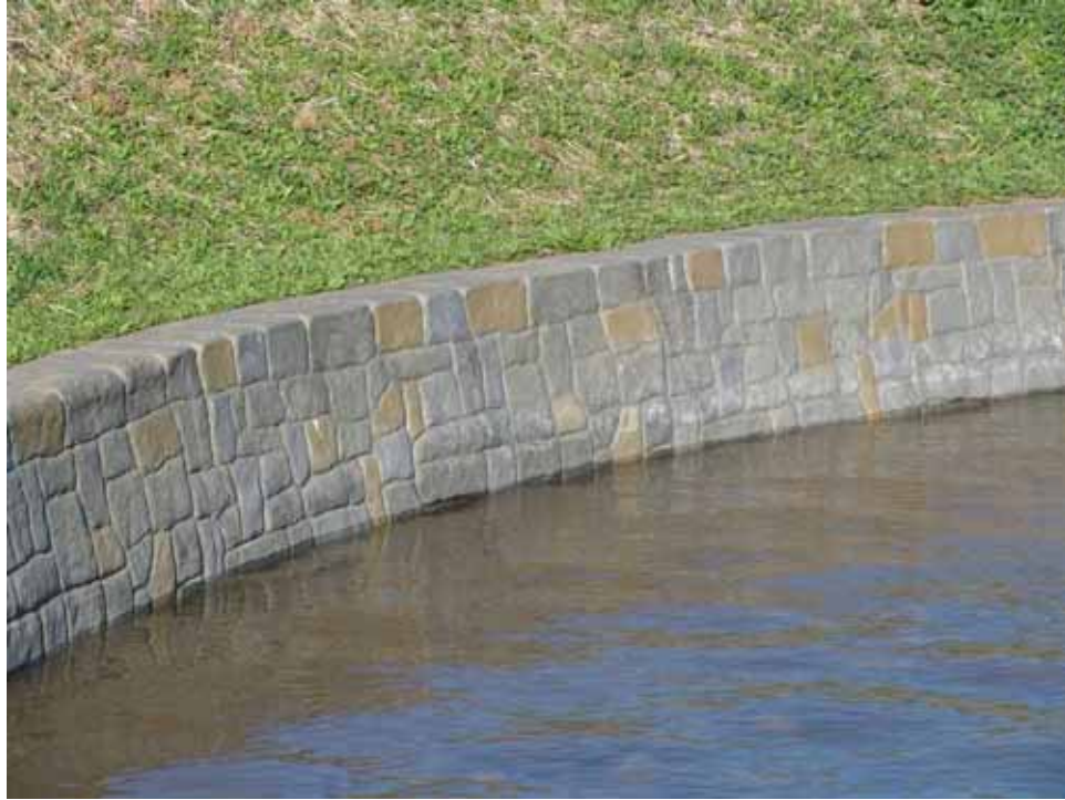
Waterside bulkhead for Reflections Lake in Patterson, CA
