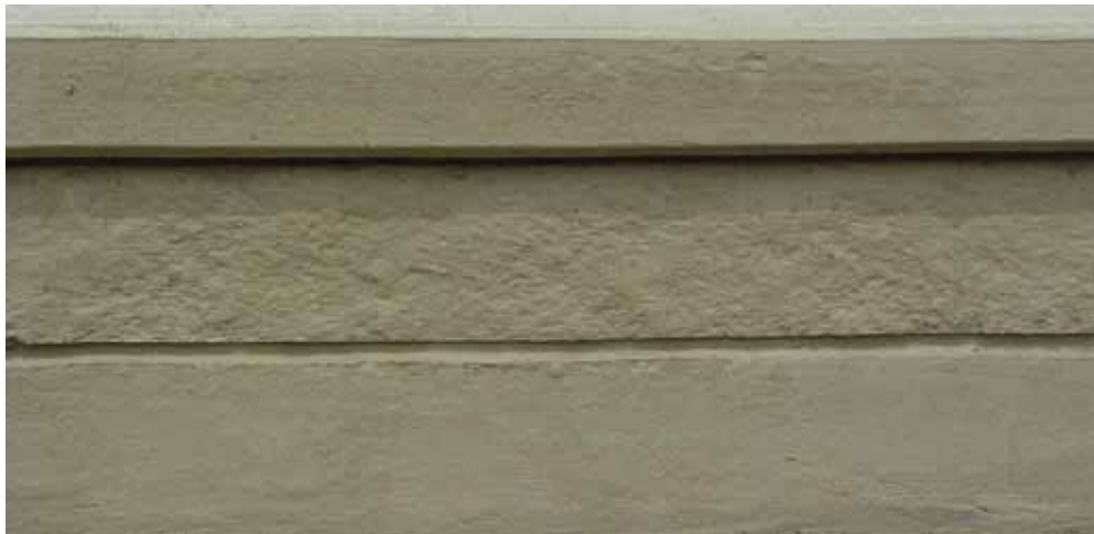
Bridge parapet on T.H. 35E in Ramsey County, Minnesota
