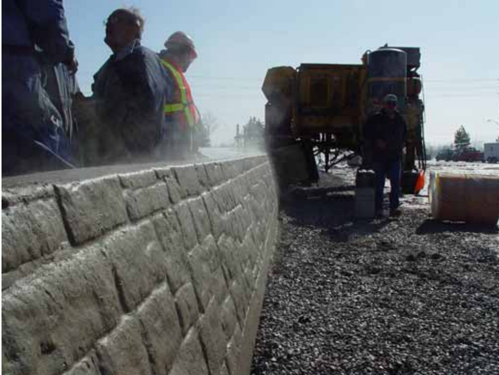
Median barrier on Niagara Hwy. 420 in Ontario, Canada
