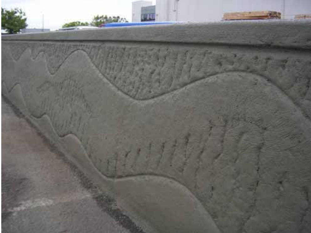
Median barrier on Interstate 5 near Los Angeles, CA
