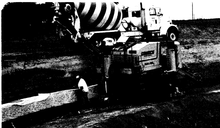
Allen & Sons only had a 15 foot (4.57 m) ledge to work on after the general contractor over-excavated the man-made lake.
