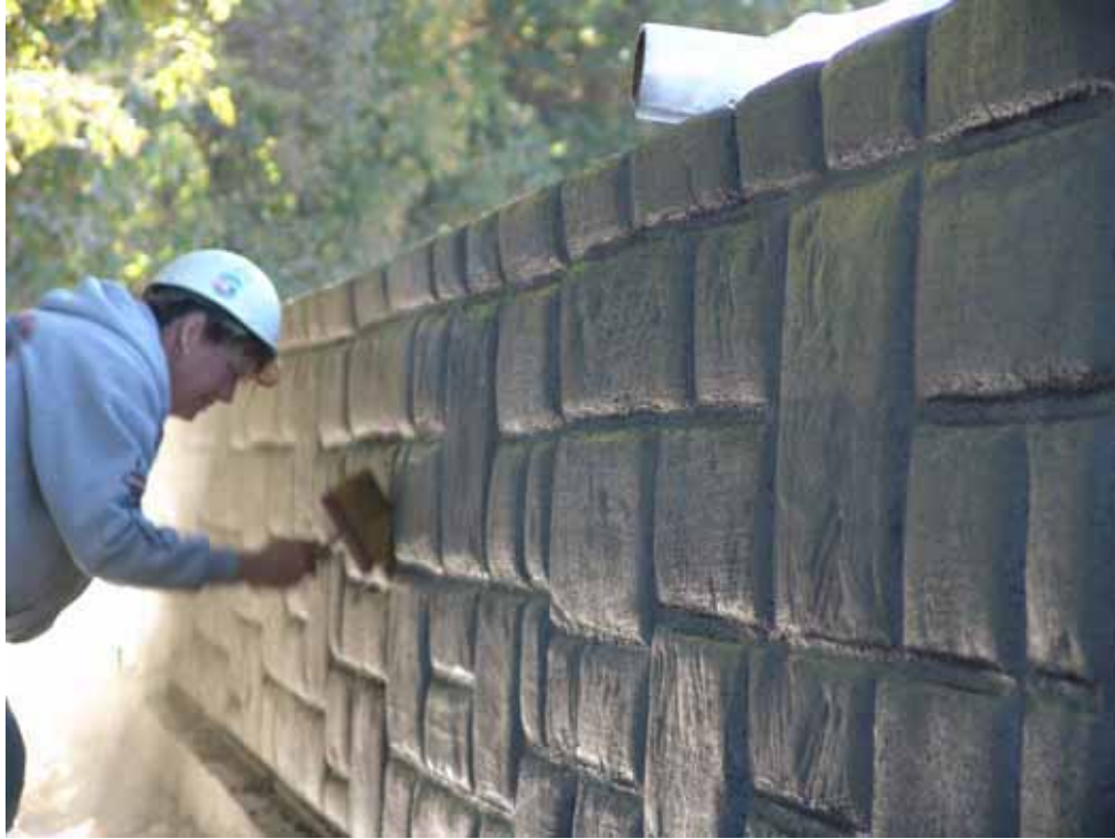
Bridge parapet on RT. 30 in Wayne County, Ohio
