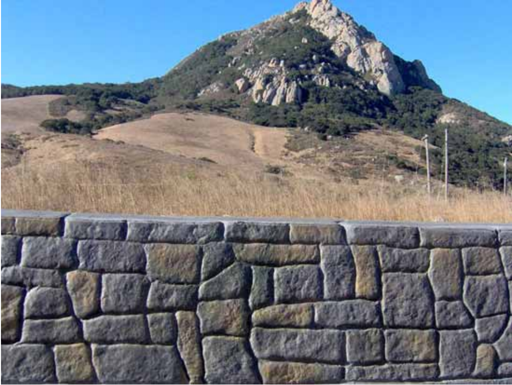
Median barrier on Hwy. 1 in Morro Bay, CA
