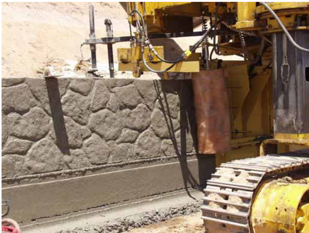
Waterside bulkhead for Sundance Lake in Modesto, CA
