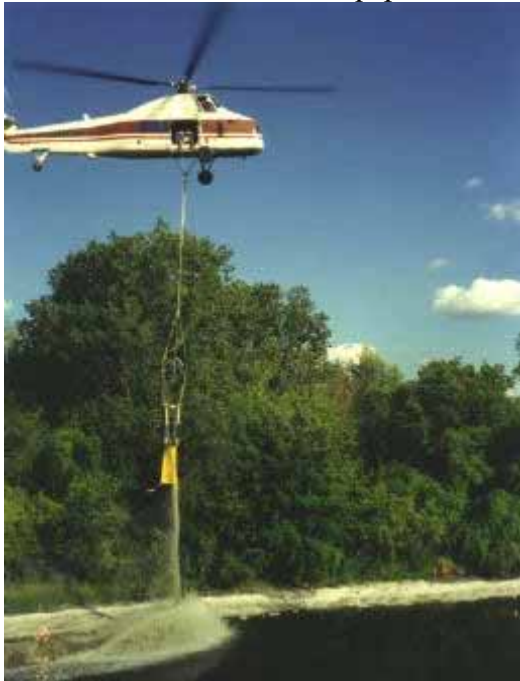
Placing Aggregate Capping Material Using a Helicopter
