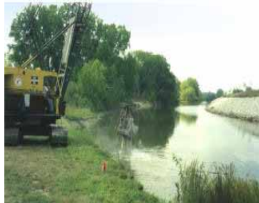
Placing Aggregate Capping Material from Shore Using a Dragline
