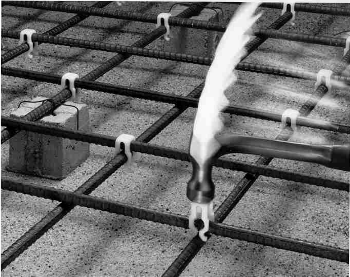
Figure 5. Example of Clip-con being installed with a hammer
