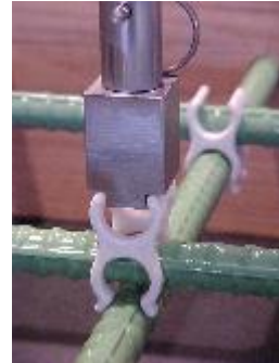
Figure 4. Kodiklip Application and Kodistik Being Pushed into Place with Kodistik Tool.
