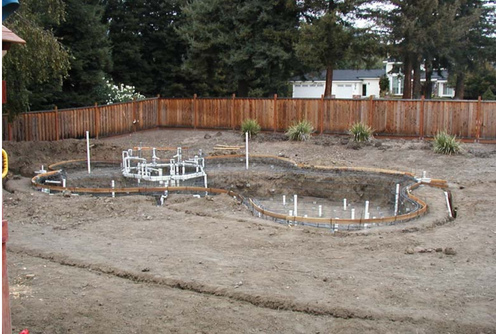
Figure 3. An Application of an In-ground Concrete Pool Tied with Speed-Clips.
