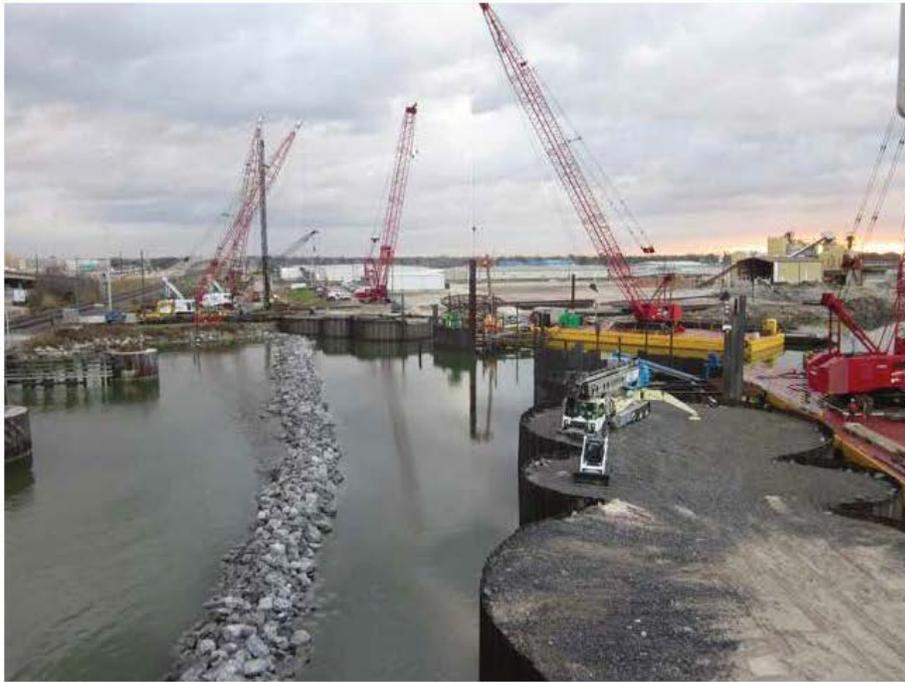
Alberici installed a temporary rock dike to sharply reduce tidal flow through the canal. The image below shows the rapid flow of the current before completion of the dike. The dike enabled use of a cofferdam. The dike was later removed for use as permanent scour protection, as shown in image below, at left.
