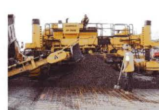
Figure 5- 1" slump concrete discharged from belt
