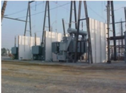
Fig 3. Three Intelli-Firewalls, each 35' x 35'
