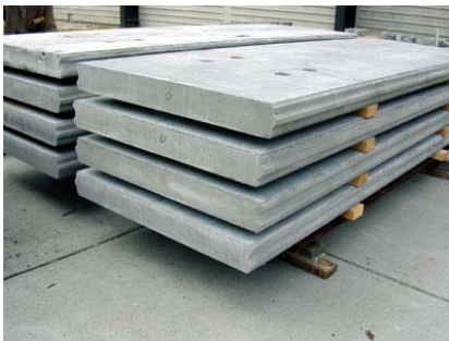
100 mm HySSIL panels prior to erection
