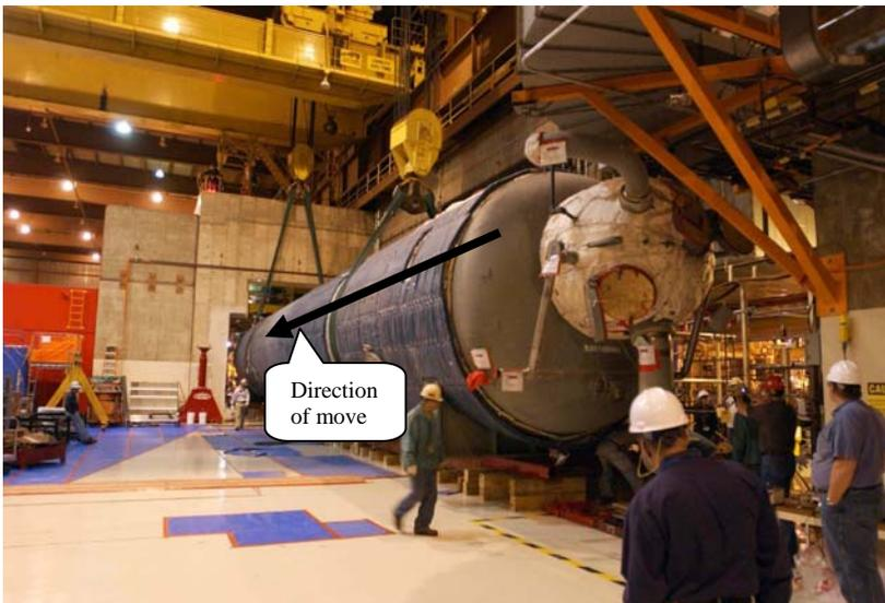
Sliding new vessel into place to 2" clearance
