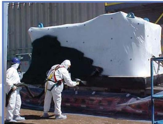
Workers used a spray-on coating that was used for over-the-road packaging for large pieces of contaminated equipment.
