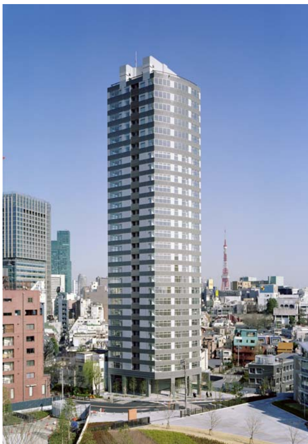
Figure 2: Glorio Roppongi high-rise residential building, located in Central Tokyo, uses ECC coupling beams in core for seismic resistance (Building height: 27-stories, 95m high; built by Kajima Corporation, construction completed in 2006).
