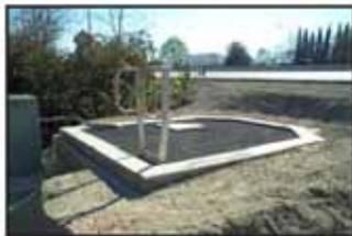
This GSRD utilizes a 3 mm (0.125 in nominal) spaced parabolic wedge-wire screen. Runoff enters the device and flows into a trough where larger gross solids settle out and the runoff is distributed. The distributed runoff flows over weirs and falls onto and through the screen. The gross solids are captured on the surface of the screen and slide down the screen to the storage area. Weep holes are provided to drain water between storm events.
