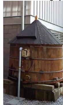
Figure 5. Pickle barrel cistern used to collect rain runoff and recycle.
