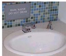
Figure 4. Rainwater collected and used in rest rooms.
