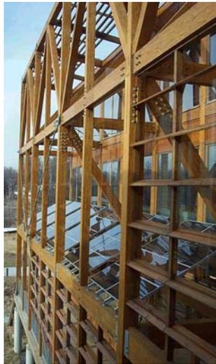
Figure 2. Photovoltaic cells on outside of structure.
