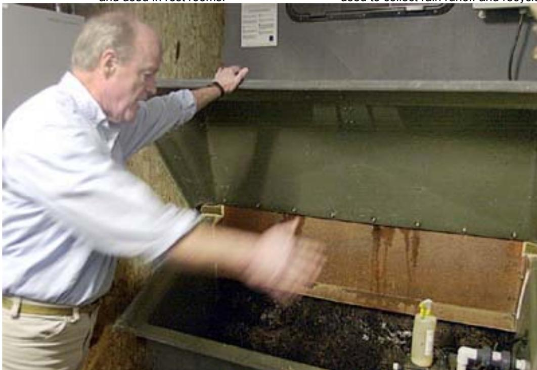
Figure 6. Ed Wintermute shows off the workings of the composting sewage system at Chesapeake Bay Foundation's Phillip Merrill Environmental Center. (photo Bill Clark / Scripps Howard News Service)
