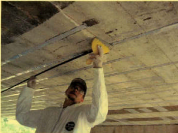
Structural Strengthening of Posted Bridge - Martin Spring Bridge in Missouri
