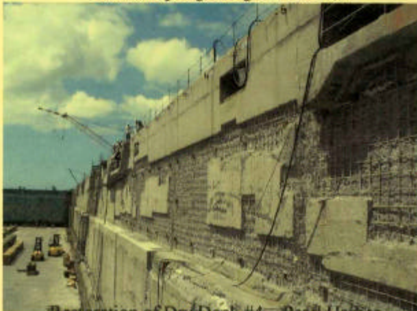
Restoration of Dry Dock #4 - Pearl Harbor
