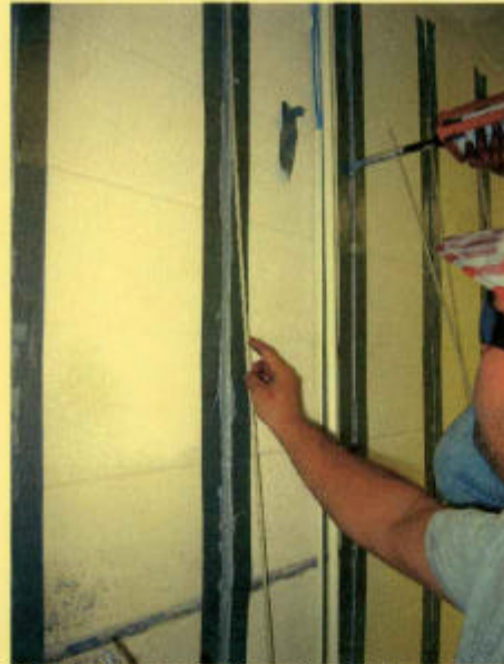
Seismic Strengthening of existing masonry
