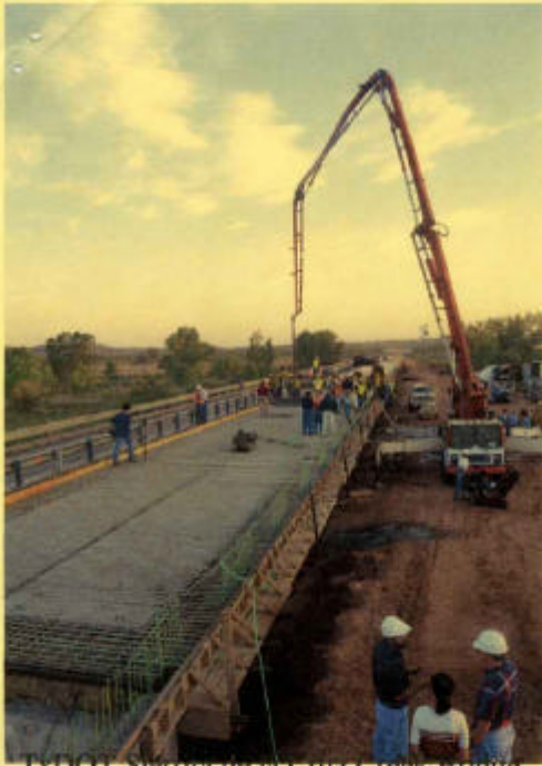
TxDOT Sierra de la Cruz Creek Bridge
