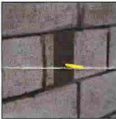
Causes no damage to the face of the block and requires no patching of block as with the plywood/nailing method of forming clean-out covers.
