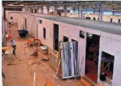
The construction of modules takes place indoors under controlled conditions.
