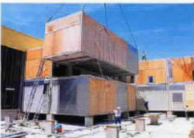
Modules are set with a pace of 4- 6 per day. In a few days to a week or two the entire building is installed at the final site.
