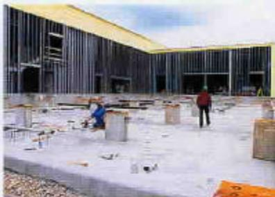
The modular plant sits on a simple foundation that has been prepared in advance by the Client.
