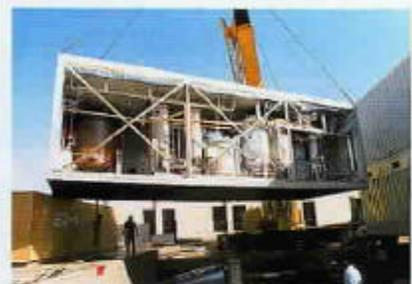
The modules are lifted in place with all equipment pre-installed. Each module weighs 15-35 tons.
