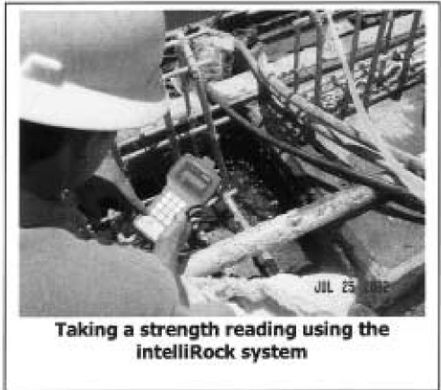
**Taking a strength reading using the IntelliRock system**
