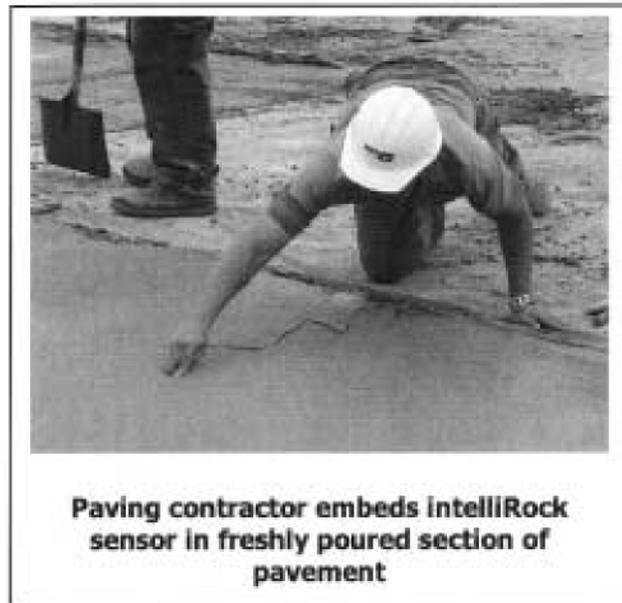
**Paving contractor embeds IntelliRock sensor in freshly poured section of pavement**
