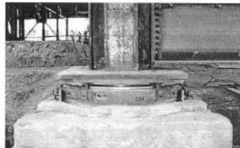
SF Airport Terminal Installed Bearing
