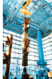
In SMART Construction, the building core and shell are assembled floor-by-floor from a covered, self-elevating construction platform that provides safety screens, scaffolding, and weather protection. As each floor is completed, computer controlled jacks lift the work platform to the elevation of the next story in about 90 minutes. Even at the 20th floor, construction workers operate in a "ground-floor" environment of improved safety, accessibility, and efficiency.
