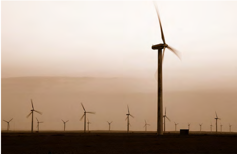
Photo: The Existing Wind Farm at Zafarana
